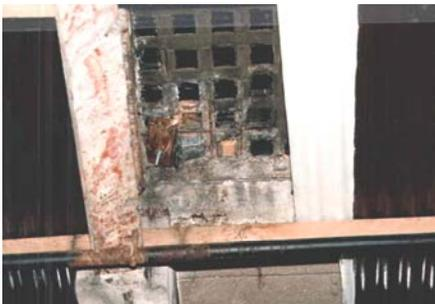
*The infrastructure of one of the city's oldest and most historic districts is collapsing. Basements of historic buildings extend out under the sidewalks on Broadway, which are in poor shape due to years of water seepage and damage to structures and infrastructure underneath the sidewalks.*
